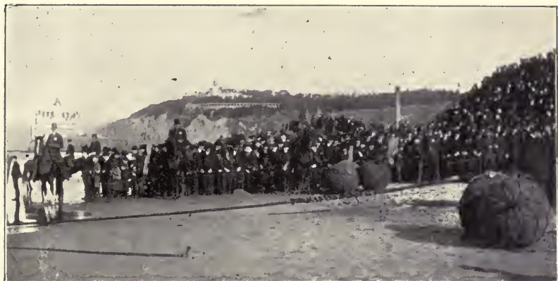
Bringing the cable ashore at San Francisco, Cal.
